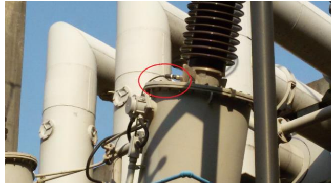
Fig. 4. Detail of adapter installation on the 230 kV bushing capacitive tap to monitor their capacitance and tangent delta.
