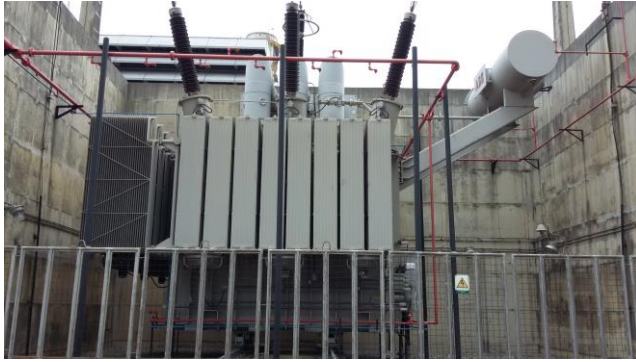
Fig. 3. One of the 225MVA, 18/230 kV step-up transformers
