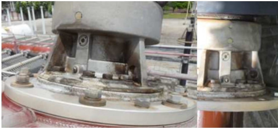
Figure 06: Cemig's team replacing the defective bushing.
